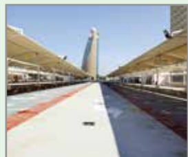
Exterior Intermediate and Exposed Decks (Car Parks Exterior, Ramps, Parking Bays)
