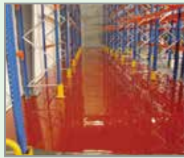
Racking Sections (Warehouses)
